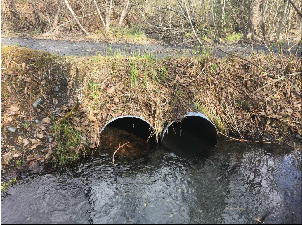
Figure 5. The Old Corbin Creek culverts on the ALPETCO trail system.
